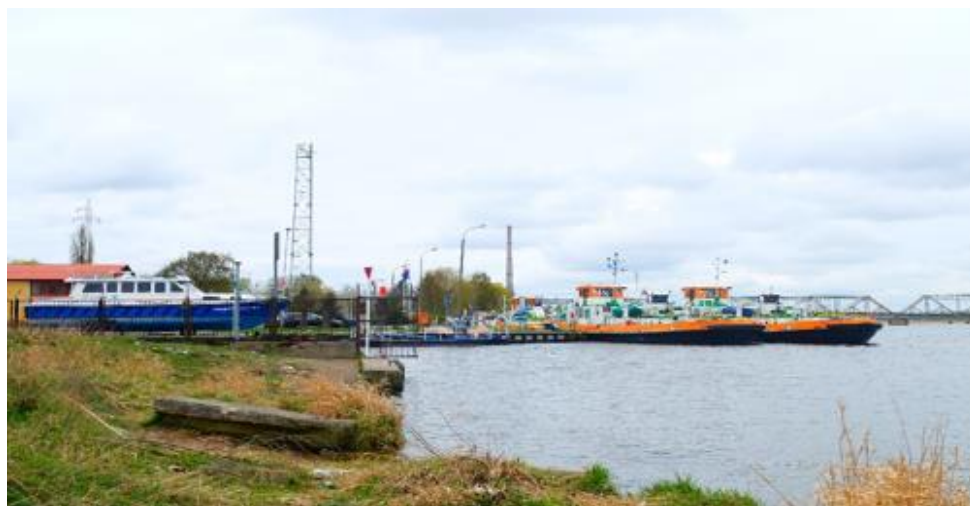
Icebreaker base, ul. Karpią in Szczecin – present condition, a view from plot No. 7/16
